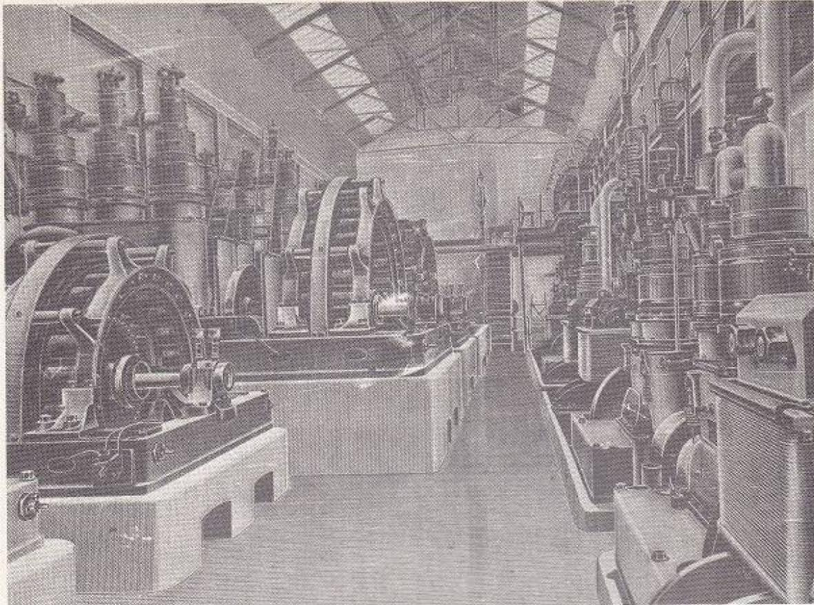
This print from *The Engineer* of 1894 shows the first Bristol public electricity supply plant as installed in 1893.
