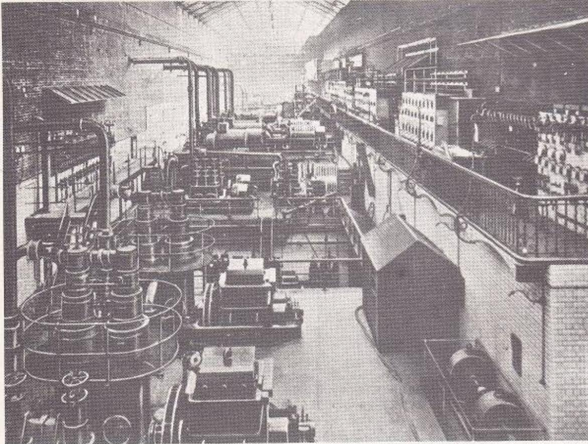
The Willans engines in the foreground were installed in 1902 and the turbines in the background were added after 1904.
