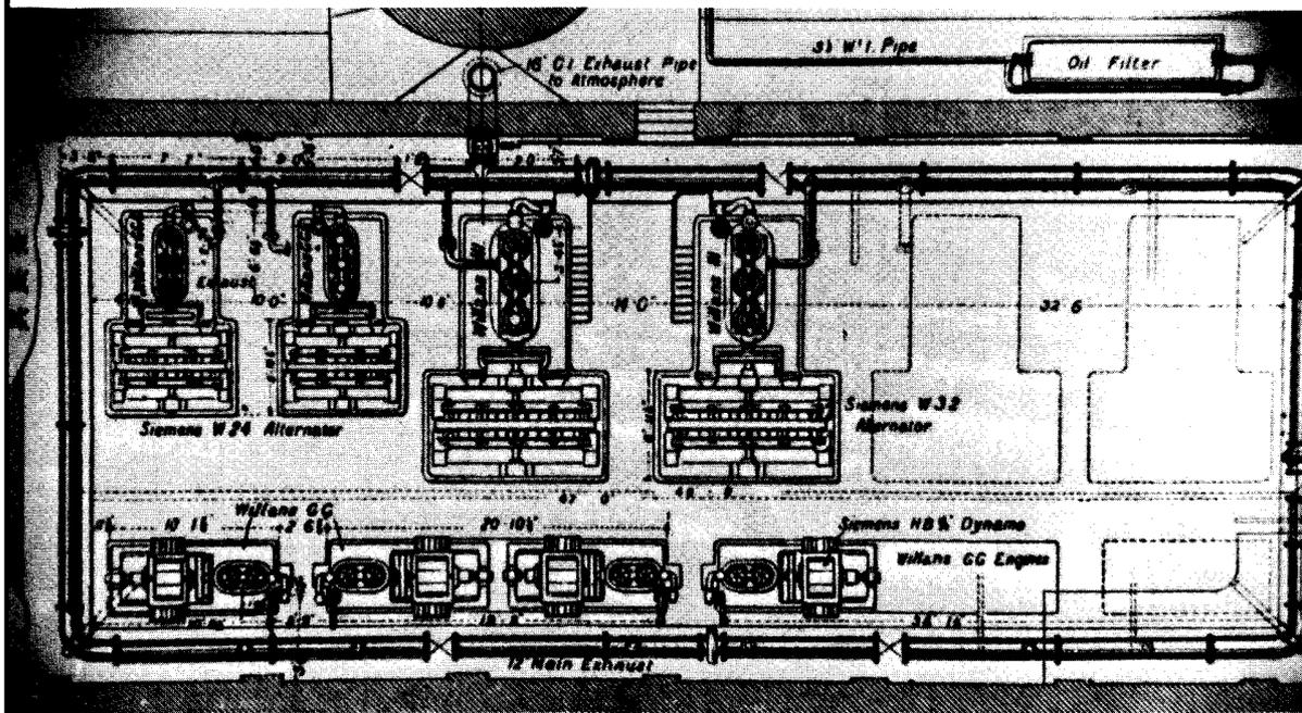
Temple Back. Plan of the first power station as in 1893, with provision for extension in the first stage. There was a second stage extension to the right beyond the condenser well. The first of the twin stacks is at top centre, and the exhaust steam ring main is shown going round the plant delivering to the condensers (right) or to atmospheric exhaust beside the chimney.
