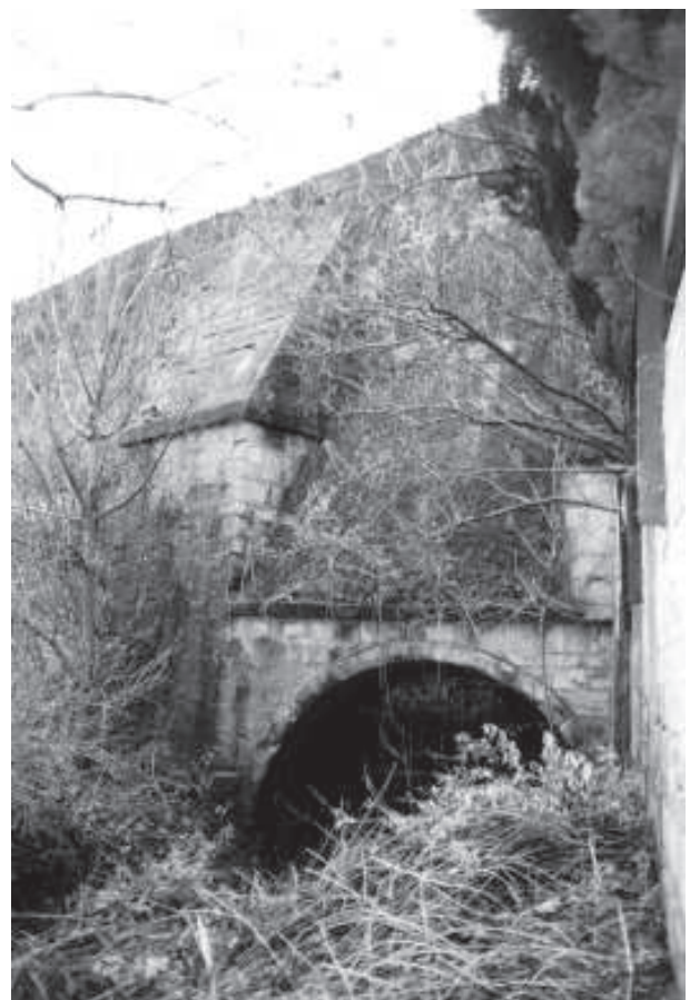
Plate 2 North portal of Entry Hill Viaduct, Bath
