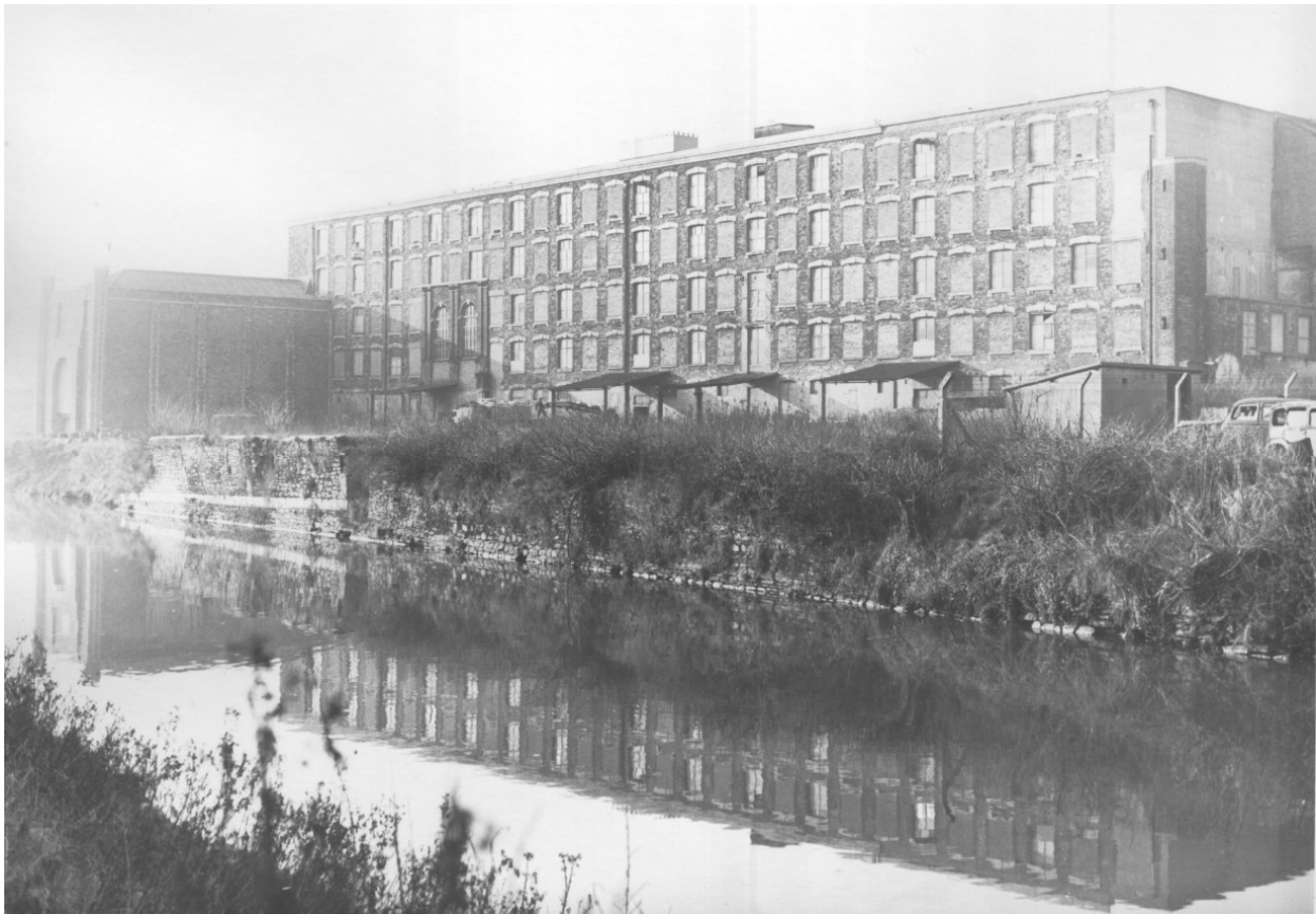
Plate 2 General view from the Feeder Canal in 1965
