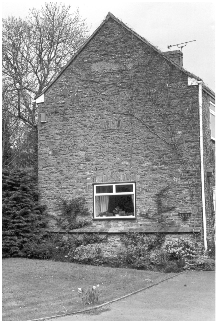
Plate 7 Bob wall of engine house (now cottage) at Yate No 2. Note arch and higher opening S. Grudgings
