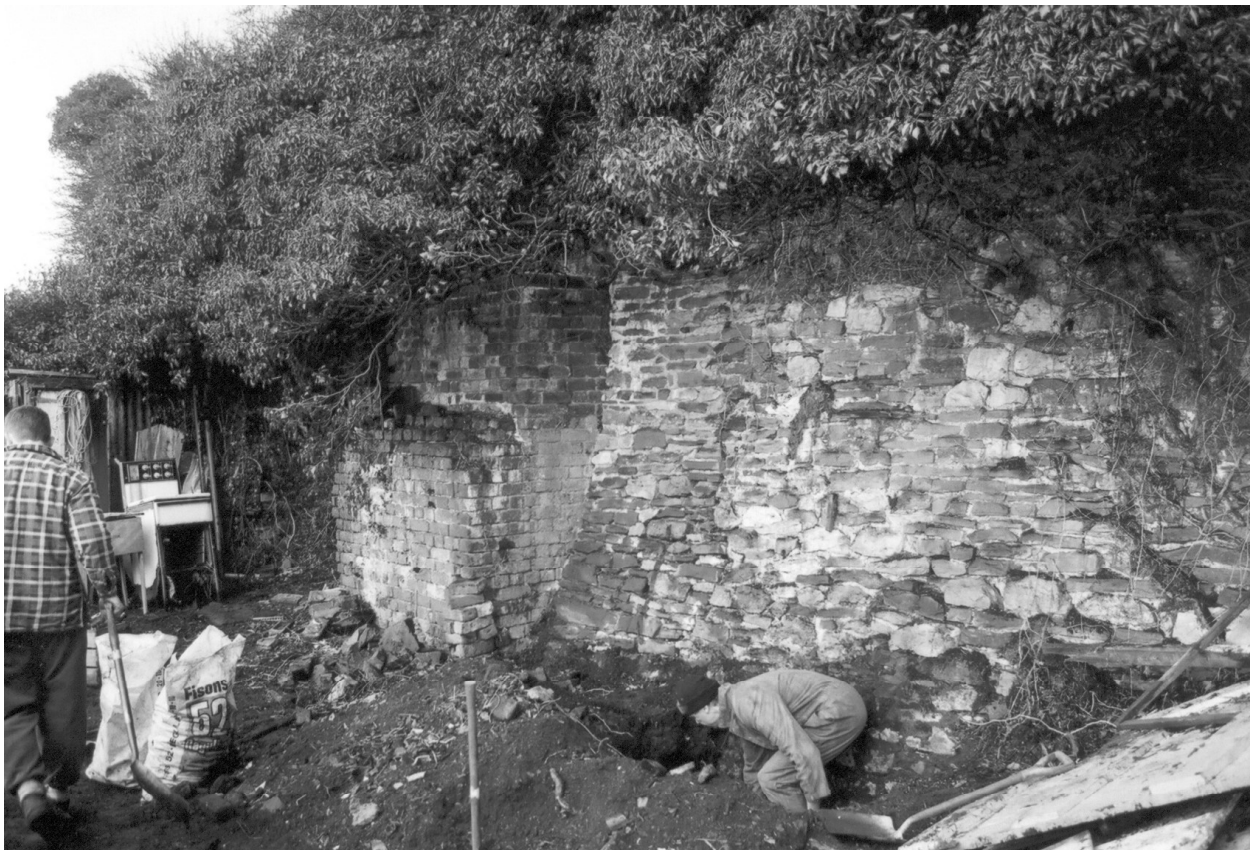
Plate 6 Excavation at Yate No 1, December 2001 alongside heapstead wall S. Grudgings
