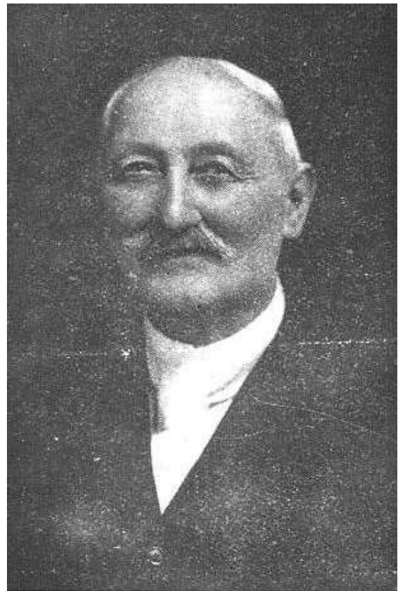
Plate 2 Henry Collyer Massingham South Western Electricity Archives
