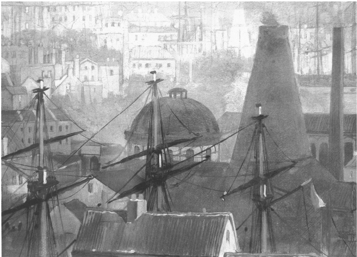
Plate 1 The original domed gas-holder of the oil-gas works on Canon's Marsh is shown here in a in detail taken from William Muller's painting of Bristol viewed from Clifton Wood, 1835. The retort house and chimney is partly hidden behind the cone of the Limekiln Lane glassworks, and in front of both are the masts of a ship berthed in Lime-kiln Dock. Bristol Museum and Art Gallery
