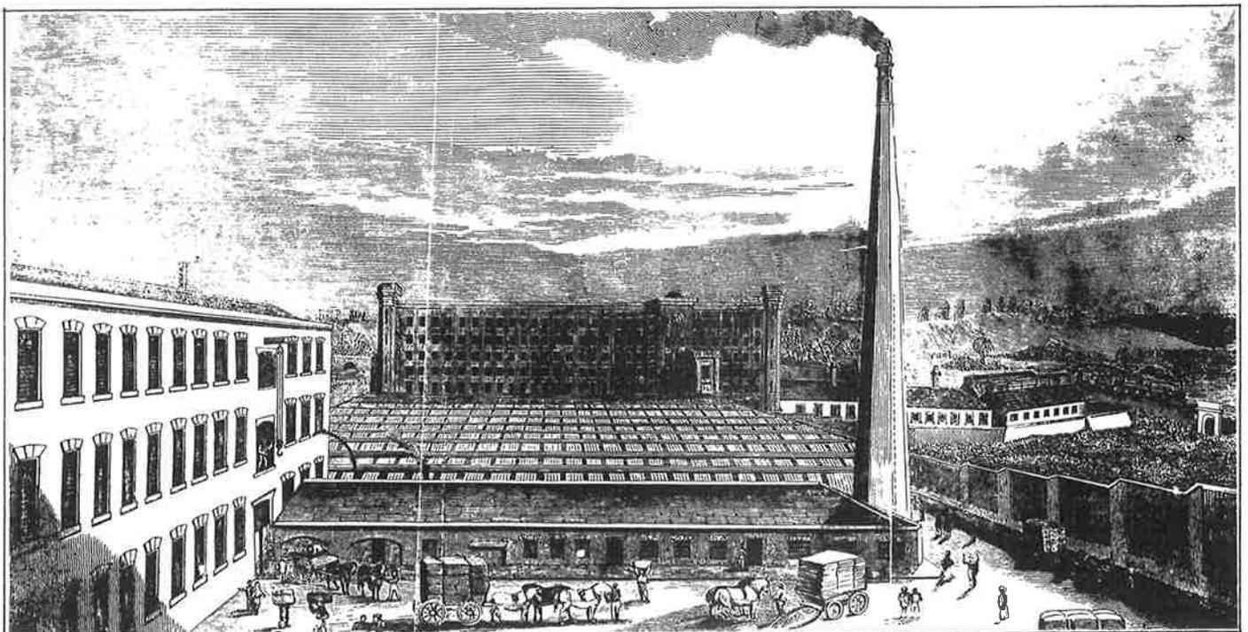
The Great Western Cotton Factory on the northern side of the Feeder Canal. This drawing from a book published in 1849 shows, on the left, the Fitting Shop, in the middle-ground the Weaving Room and in the background the Spinning Mill.
