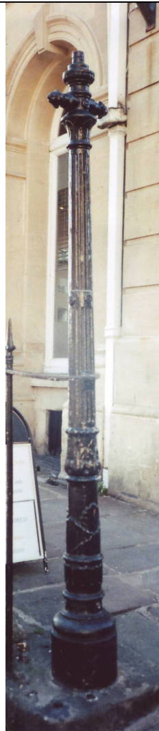
P14: experimental post: corner of Royal York Crescent Height: 7'6" Date unknown but forms part of railings. Moulded base with foliate capital. Manufacturer: unknown
