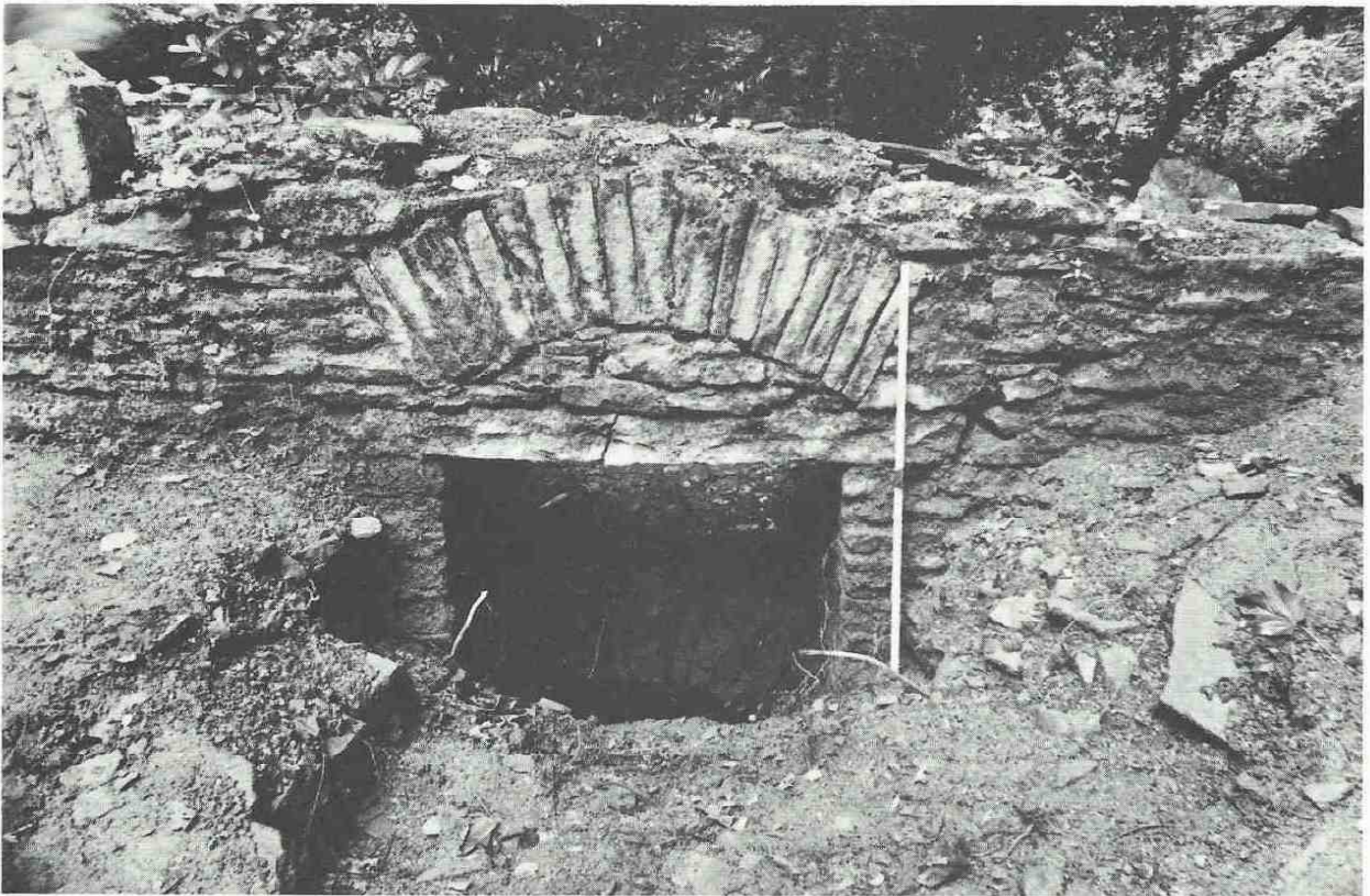
KING'S MILL The archway seen from inside the mill during the current excavations, with the bridge visible through it. The scale is a metre ruler. (Photo: John Cornwell)
