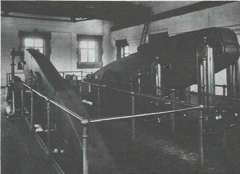
*Beams of the Watt engine at Chelvey,*
