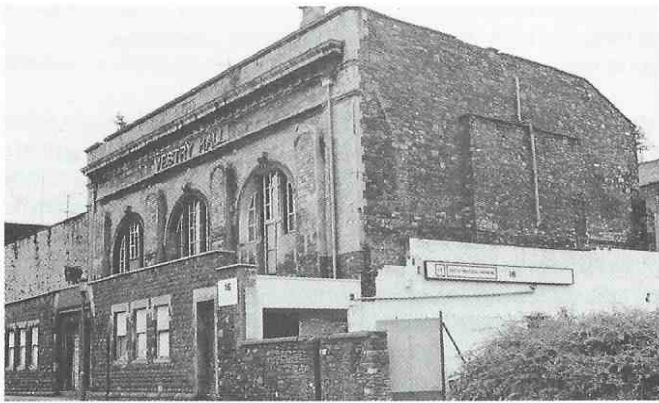
Vestry Hall, built in 1880, a cinema from 1909. 95 years old.
