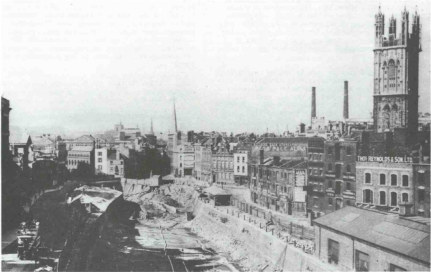
Creating Colston Avenue in the centre of Bristol by culverting the River Frome in 1892. The warehouse immediately to the left of that occupied by Thos. Reynolds and Son Ltd, bears the legend 'Coalbrookdale Compy. General Founders & Iron Merchants'. Photograph reproduced by courtesy of the Port of Bristol Authority.
