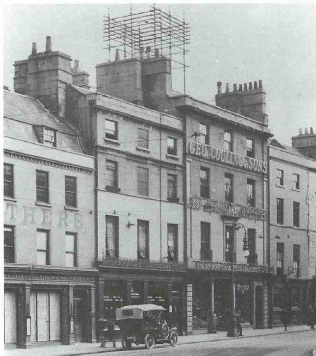
*Bath manual exchange, 11 Northgate Street, 1908, showing the exchange derrick. Photograph by courtesy of the Post Office Records Office.*
