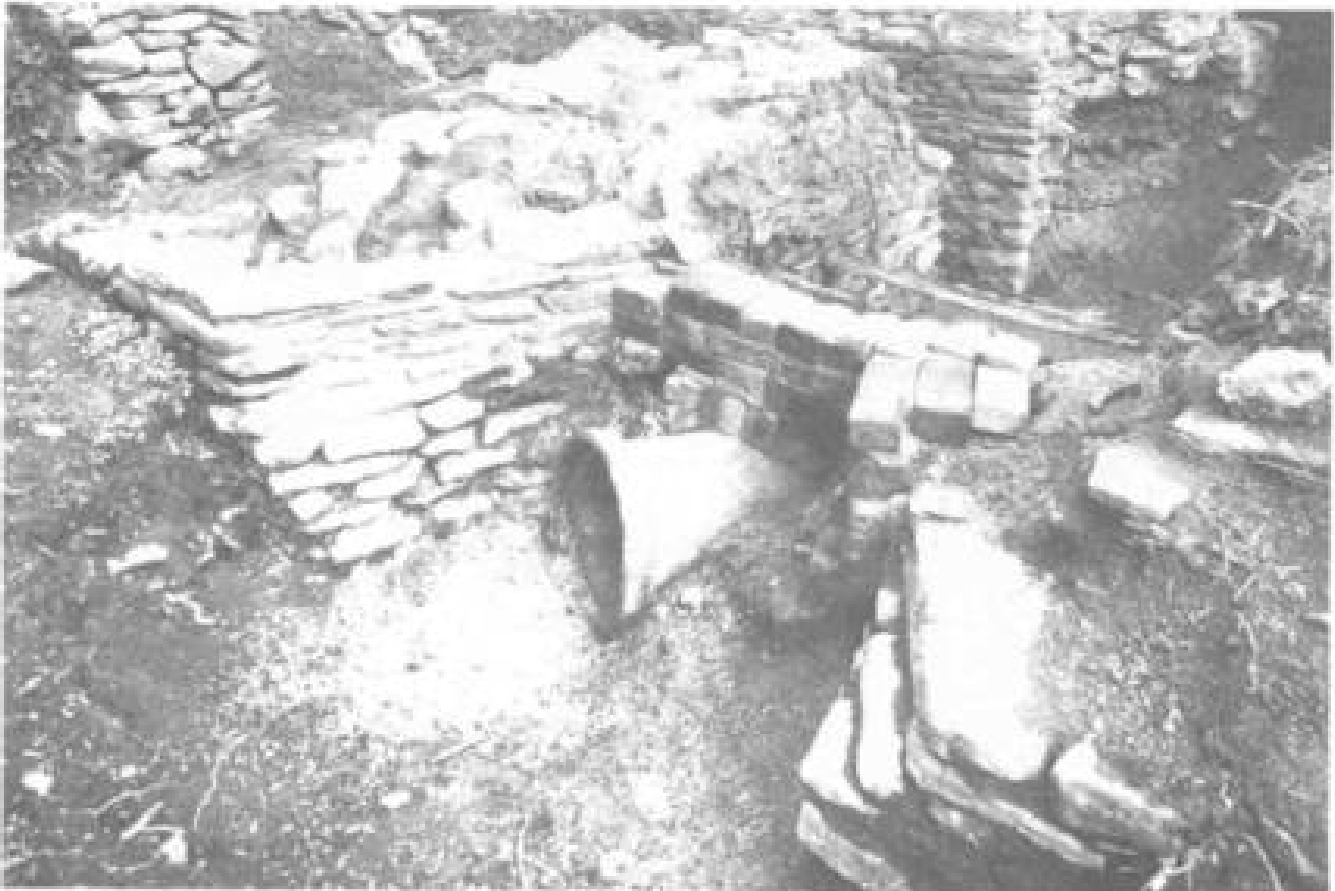
Egg Ended boiler setting, note large pipe for additional draught.
