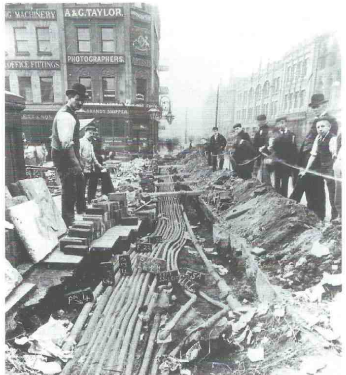
Cable laying along Baldwin Street, 1893 (SWEB Archive)
