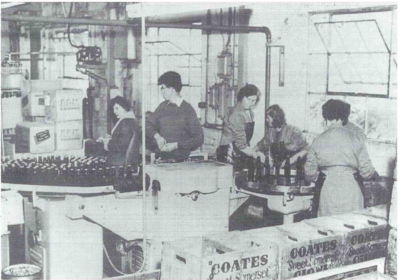
Bottling hall showing half pints being crowned
