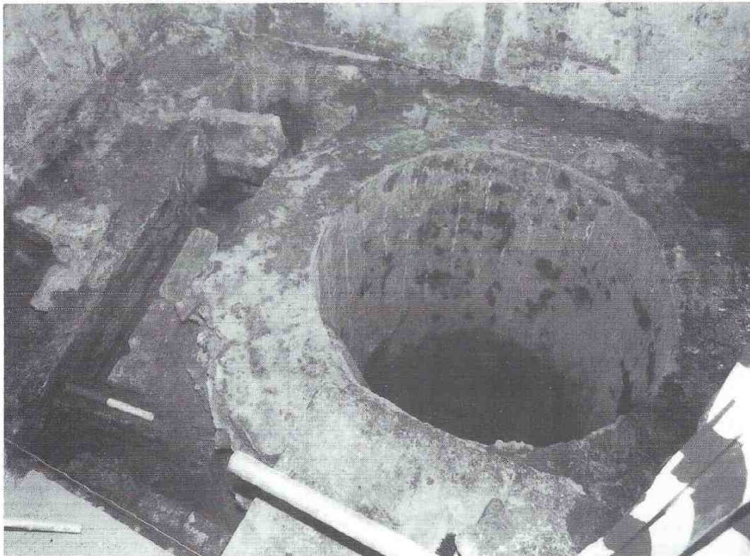
Mixing tank for the production of carbon dioxide gas
