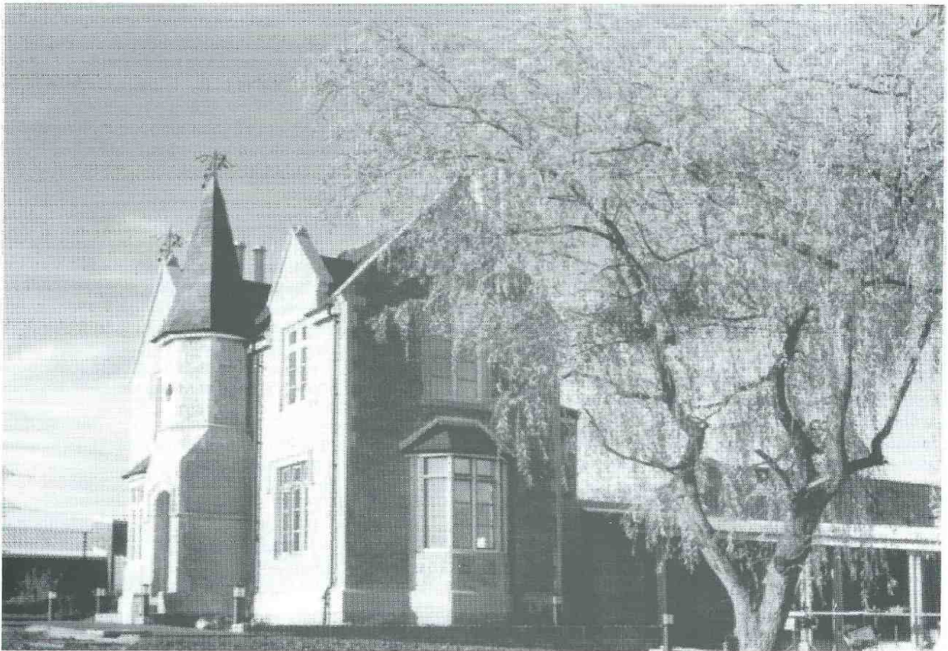
Stanley Farm fully restored.
