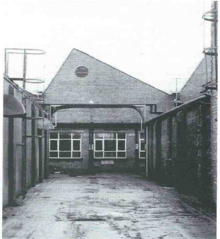
North-lit sheds (E) from west (7 October 1995).
