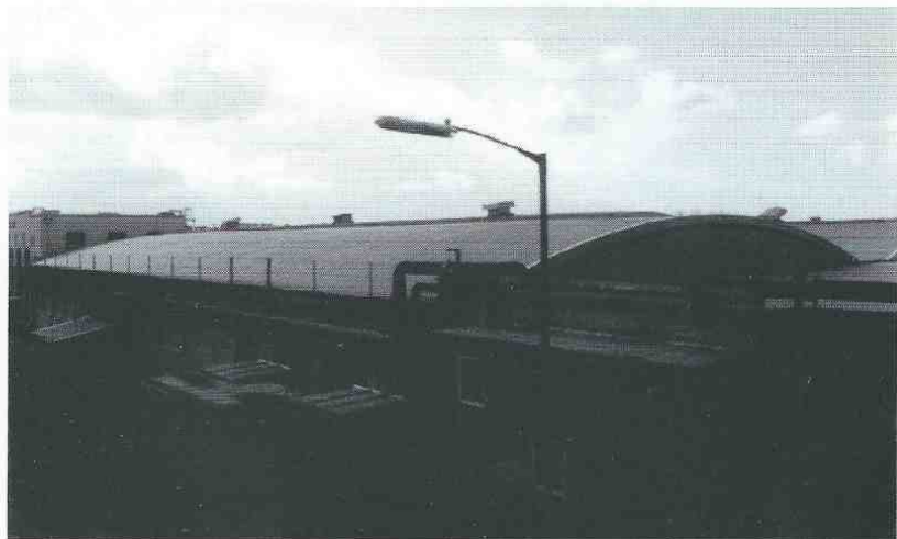
North hangar (C) from north-east, showing arched roof (15 March 1995).
