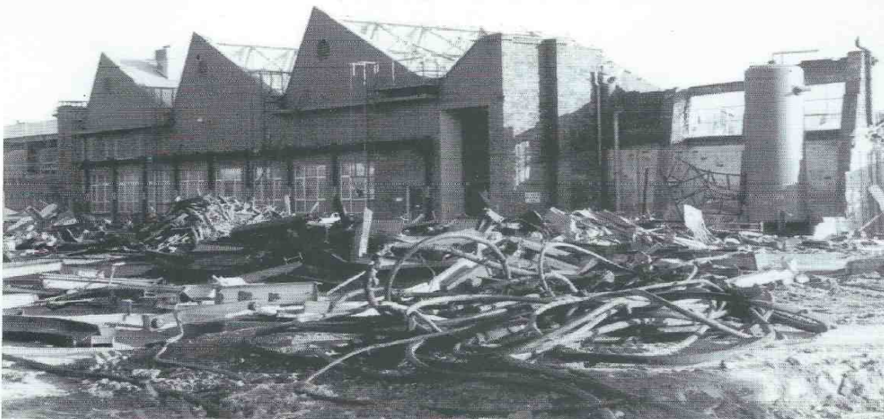
North-lit sheds (E) from south-west during demolition (2 November 1995).
