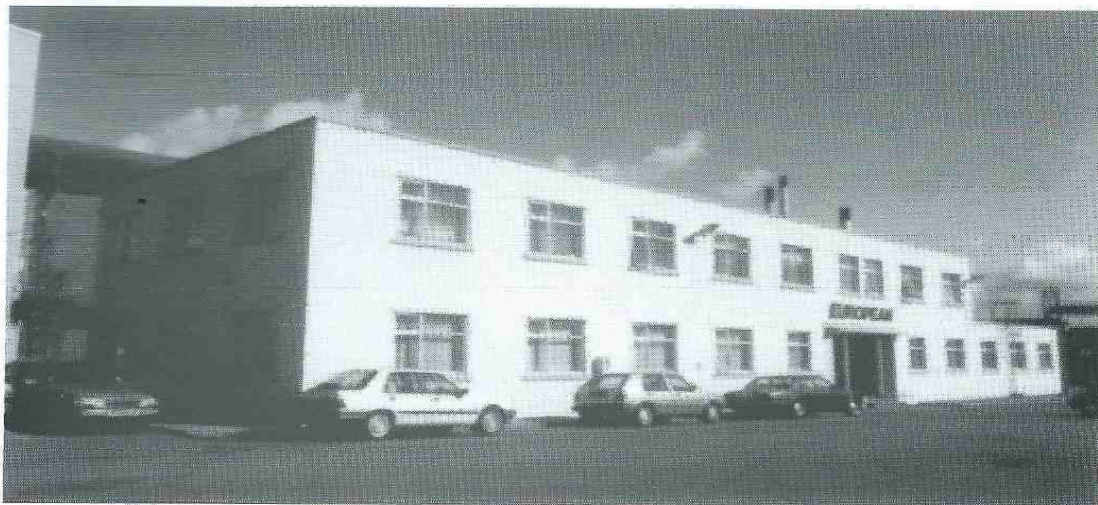
Flight operations offices (Q) from south-west (15 March 1995).
