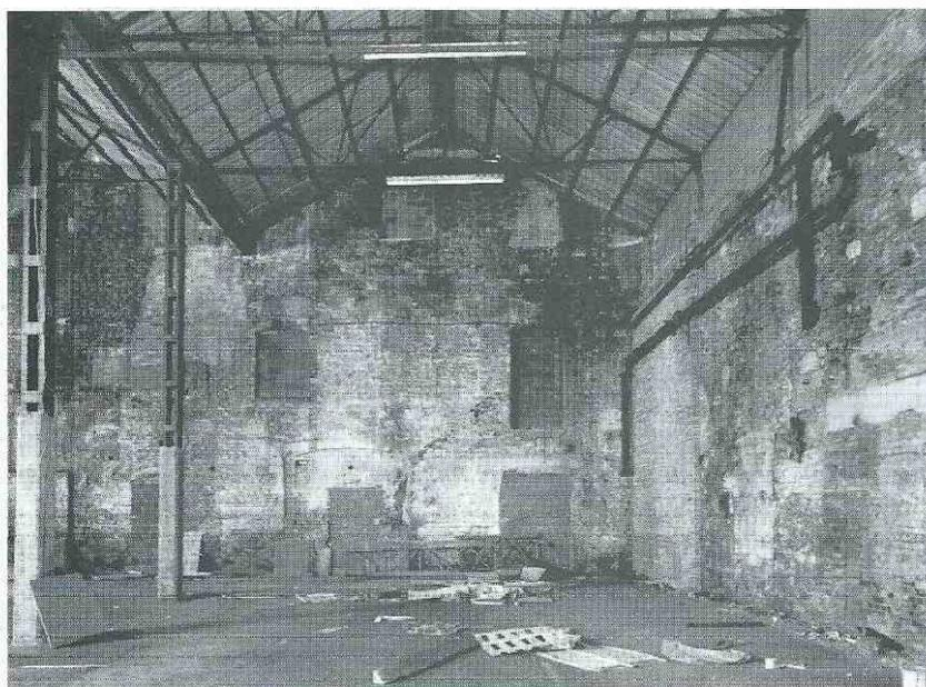
South wall of the engine house cross range showing its intersection with a partially rebuilt section of the west wall [BB96/5263 - Crown Copyright, RCHME]
