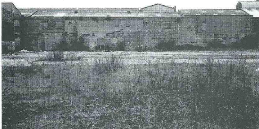
Queen-post trussed roof over the northern end of the c1837 erecting shop range. The scarred section of wall on the left of the picture marks the position of the original gable end wall. [BB96/5241 - Crown Copyright, RCHME]
