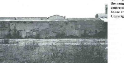
Heavily patched east wall of the original erecting shop. The gabled roof behind the range closest to the camera near the centre of the picture is part of the engine house cross range. [BB96/5273 - Crown Copyright, RCHME]
