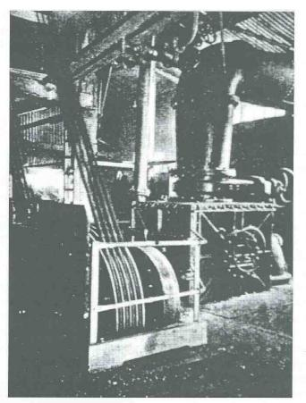
The water turbine built by Messrs King and Co of Nailsworth, Gloucester
