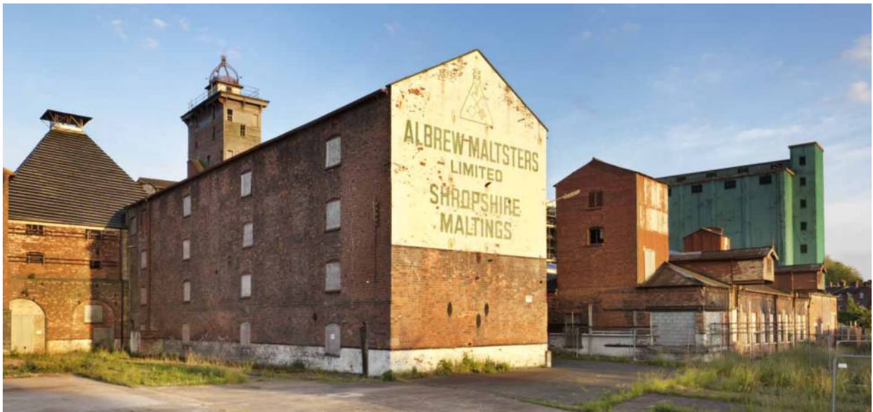
FIG. 7. Supported by the Heritage Lottery Fund, the master-plan for Shrewsbury Flaxmill Maltings is being reviewed to work up a viable scheme for the repair and use of the main mill. A major monograph shedding new light on this internationally important site is also being published by Historic England in November 2015 with contributions from leading experts. © James O. Davies, Historic England
