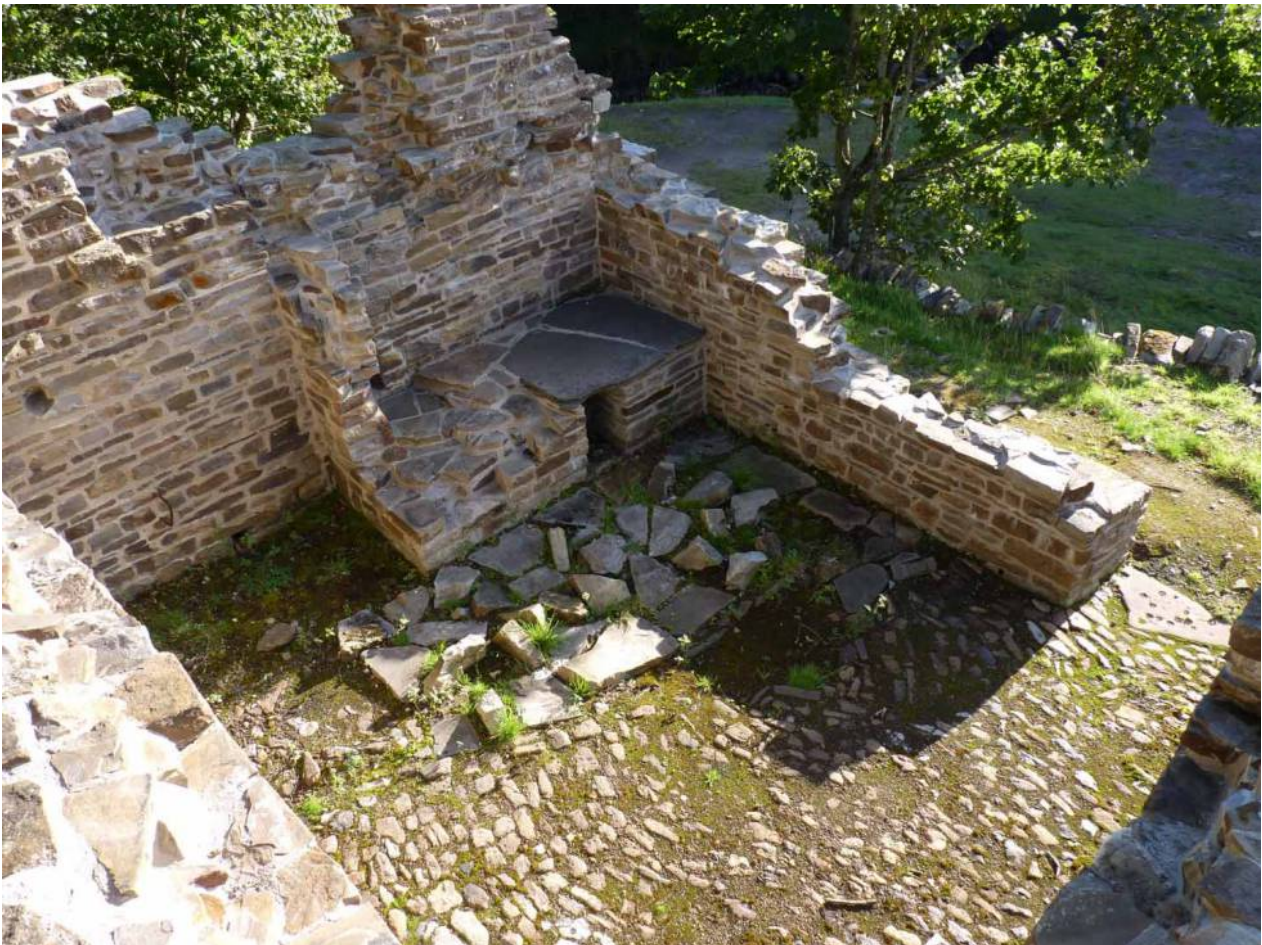
FIG. 3. Conservation works at the Low Slit Lead Mine has improved public access and interpretation, whilst enhancing the flora on this Site of Special Scientific Interest. Having been removed from the Heritage at Risk Register, it was presented with an Historic England Angel Award in 2013, see below. This image shows the repaired and conserved mine smithy. © Kevin Doonan Architect Ltd
