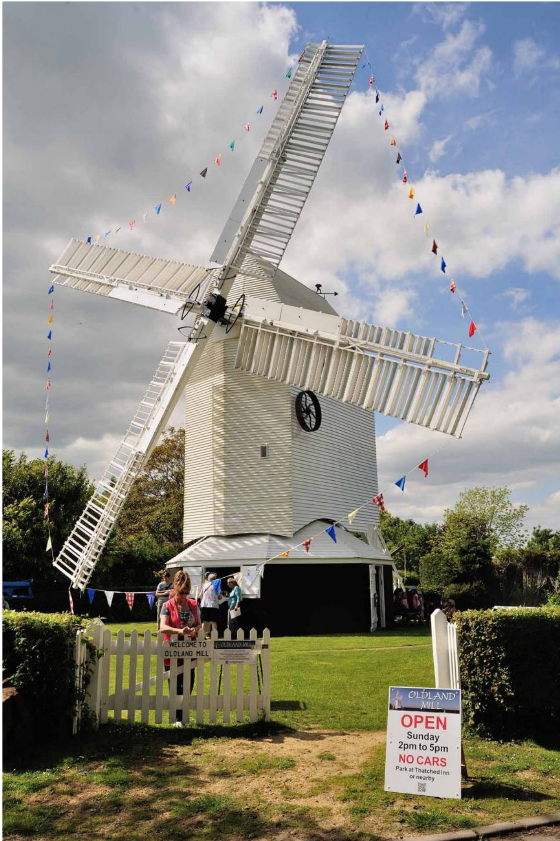
FIG. 12. The Oldland Mill project in West Sussex involved the total dismantling and restoration of the body of this Grade II listed windmill, as well as replacing all four sweeps, which took more than 30 years with over 100,000 hours of volunteer effort. Thanks to the work of the Oldland Mill Trust, it is the oldest working windmill in Sussex, produces flour once more and opens regularly as a local cultural and educational resource. In 2014 it was voted as the people's favourite for an 'Historic England Angel Award'.
