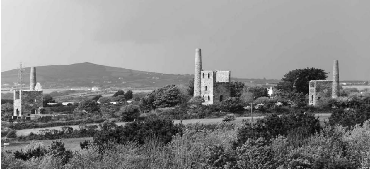
FIG. 5. Wheal Peevor, Cornwall. This is the only surviving site where the once common arrangement of three engine houses for pumping, winding and stamping can still be seen.
