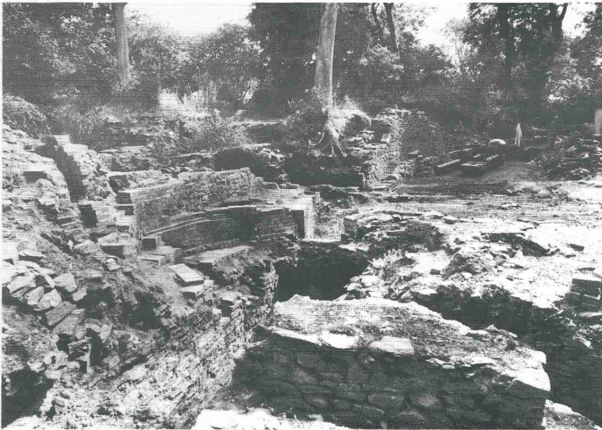
view of Old Pit site looking South from the rear of the Haystack boiler setting.
