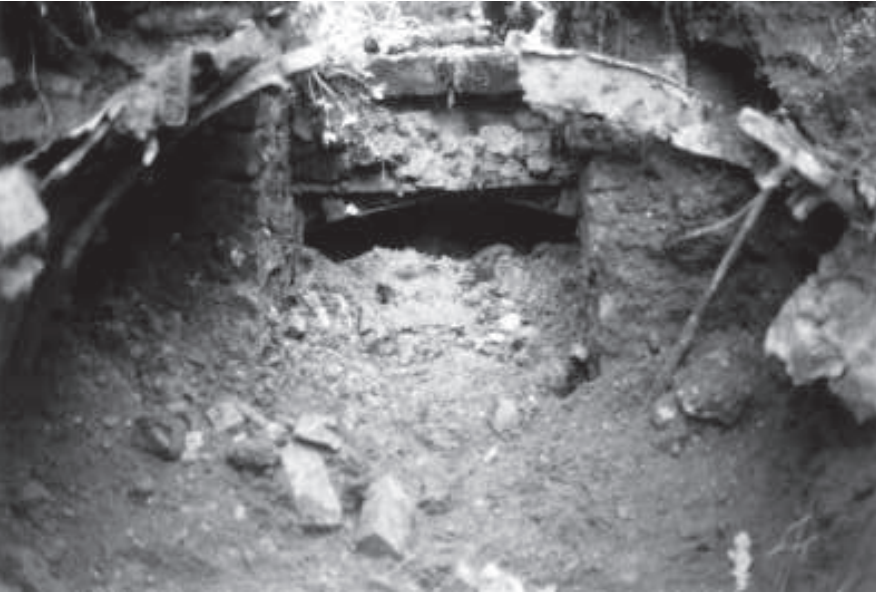
Plate 3 View through the waterwheel showing the second wheel beneath the arch
