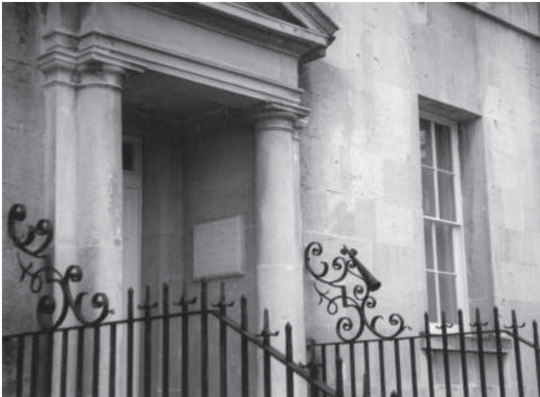
Plate 1 Snuffer for extinguishing rush torches known as link snuffers. The Royal Crescent, Bath Mike Chapman
