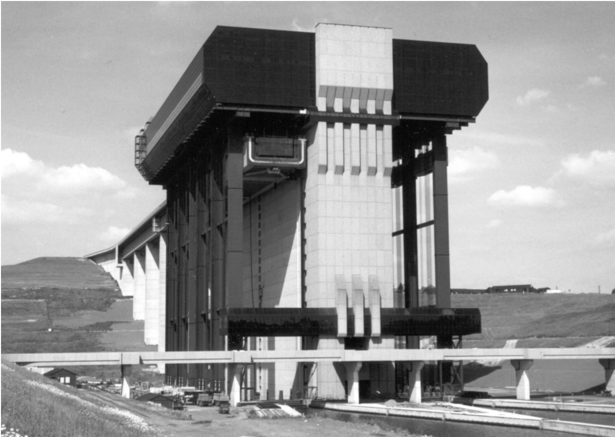
Fig. 12 Strepoy Lift nearing completion, 1999.
