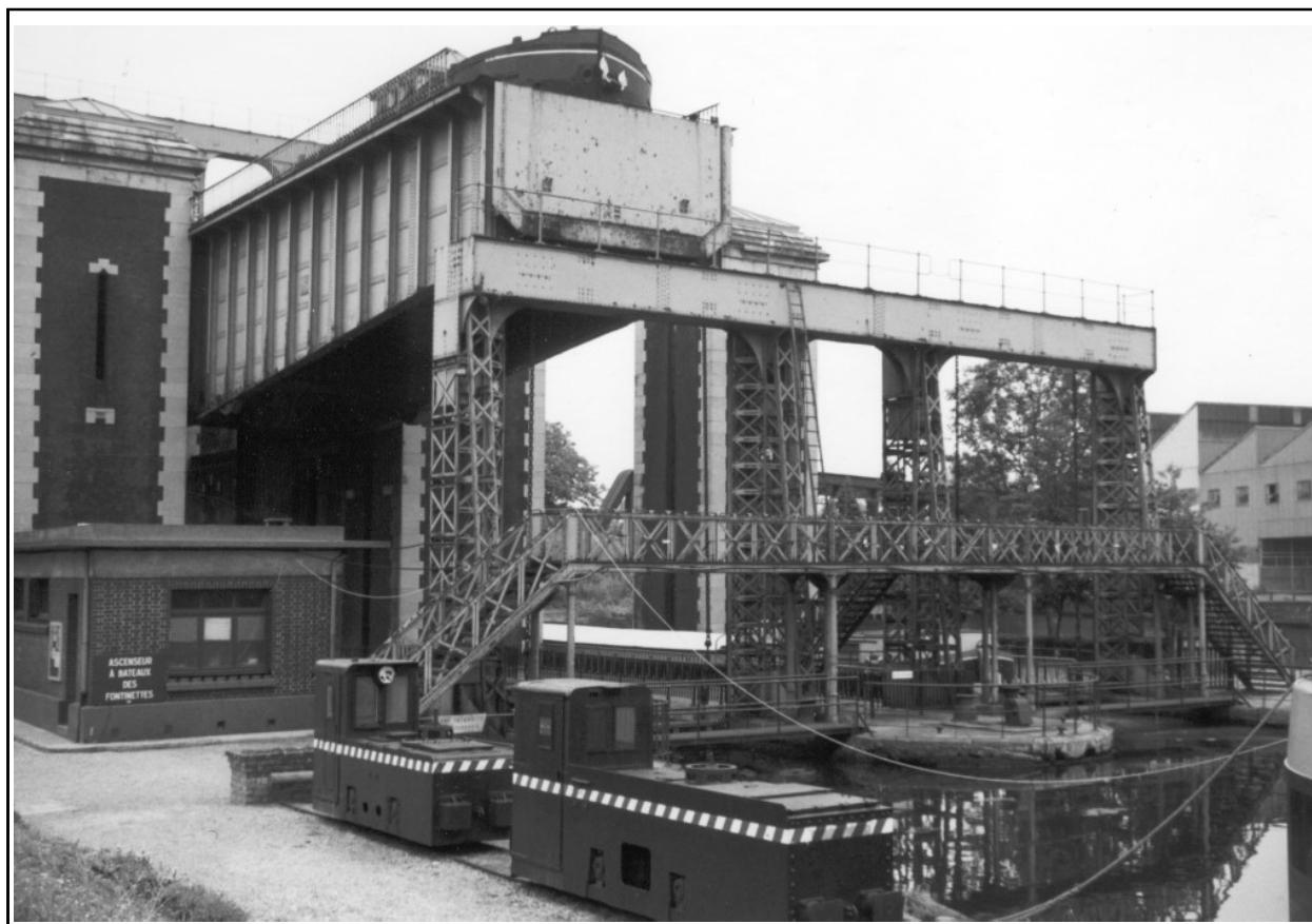
Fig. 8 Hydraulic Lift, Les Fontinettes, France, 1999. Note the boats in both caissons
