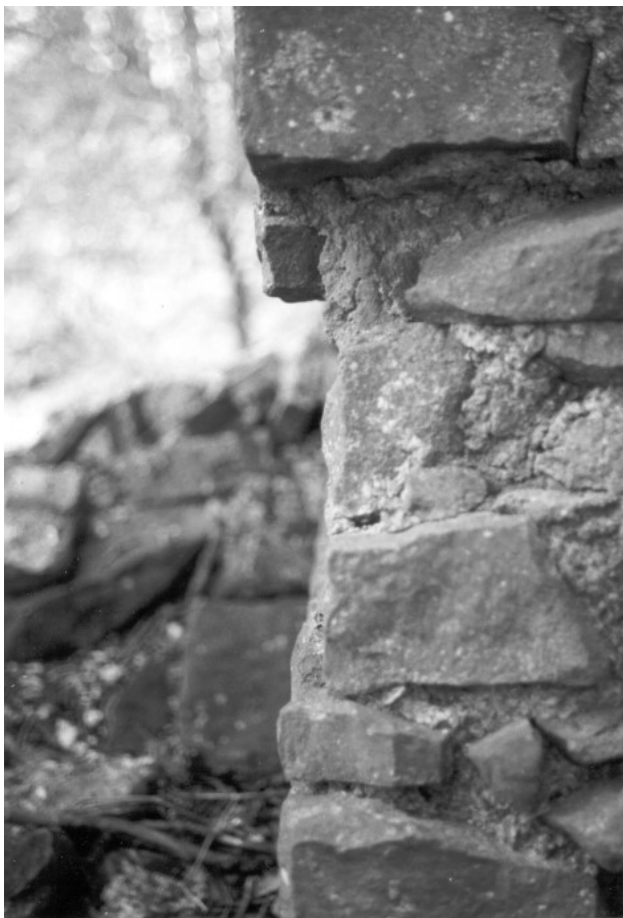
Plate 8 Curved recess in engine house wall
