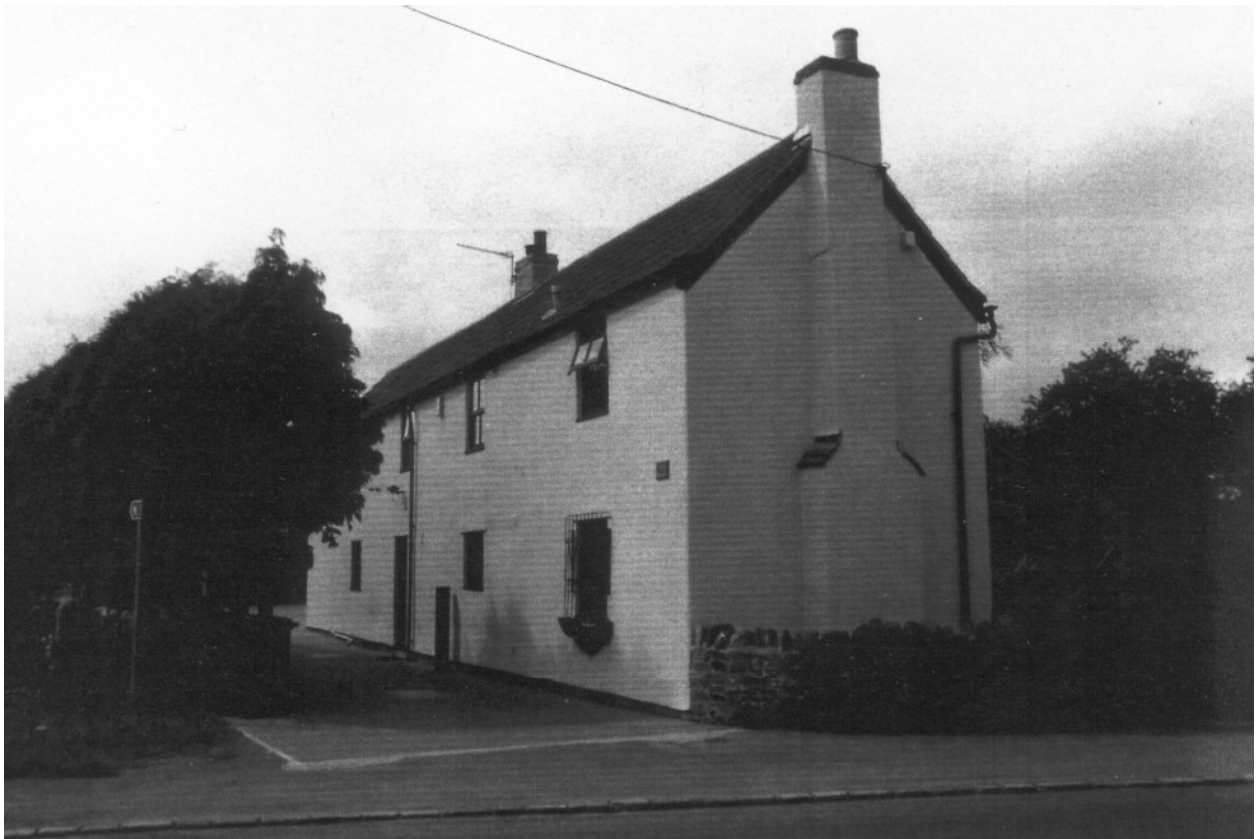
Plate 2 Holly Manor - previously called Sunnyside and Old Engine Cottage (May 1999)
