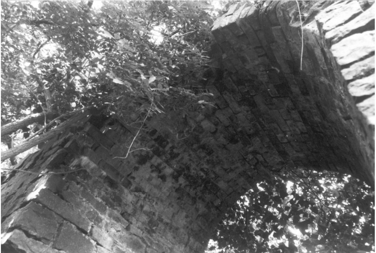
Plate 7 Arch in bob wall of engine house
