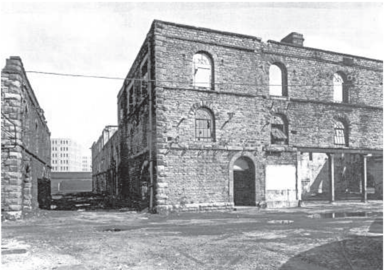
Plate 2 Retort house (south-east block), Canon's Marsh Gasworks, August 1970
