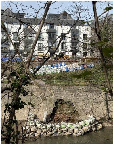
New Cut wall near Gaol Ferry Bridge – photo: Martin Booth
